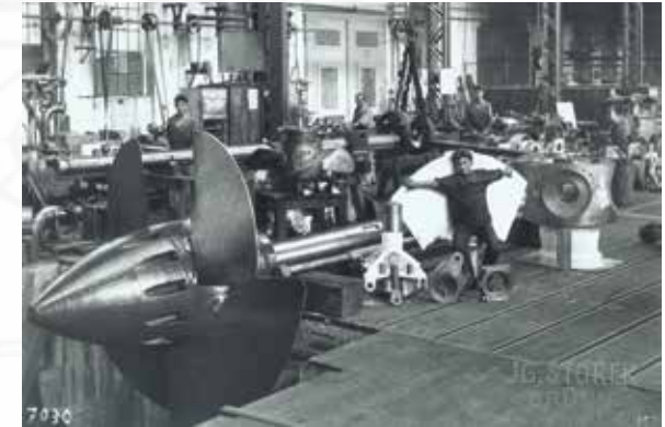
Insight into the production of Kaplan's turbines
